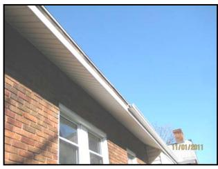
Fixing and replaces portions of gutters and downspouts are inexpensive repairs that preserves roofs and foundations.
